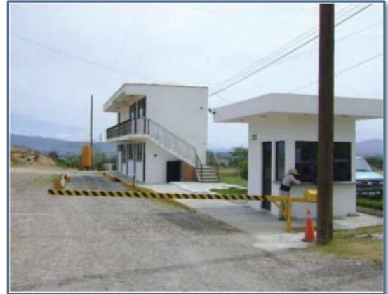
Good Practice: Secure controlled landfill with guarded access and fenced perimeter
