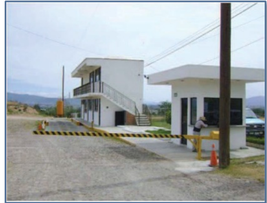
Good Practice: Secure controlled landfill with guarded access and fenced perimeter
