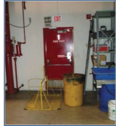
Bad Practice (IA): Fire exit is blocked by trash container and equipment
