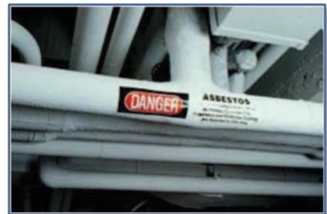
Good Practice: Asbestos-coated pipes are properly marked.
