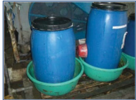
Bad Practice (IA): Secondary containment is too small for these chemical drums!
