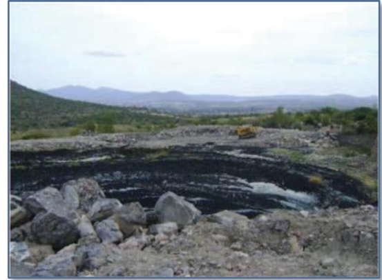
Example of a mono-fill: a sludge pit that is properly lined.
