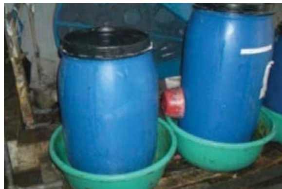
Bad Practice IA: Secondary containment is too small for these chemical drums!
