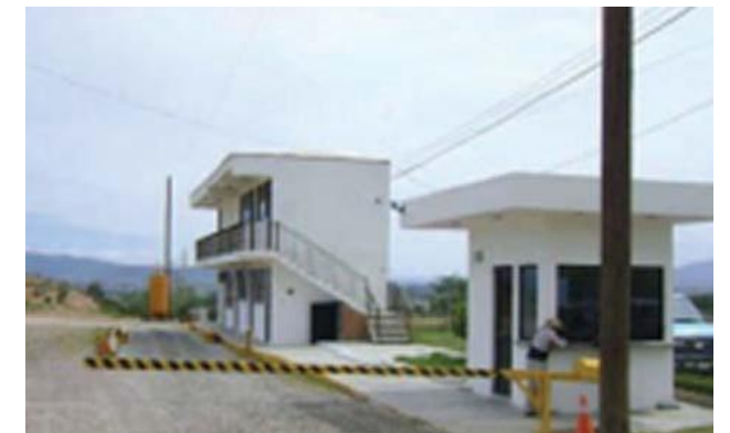
Good Practice: Secure controlled landfill with guarded access and fenced perimeter
