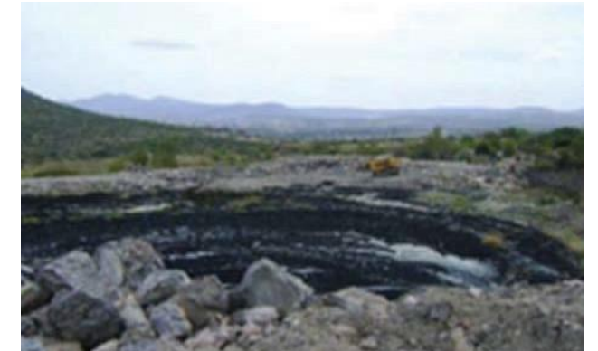
Example of a mono-fill: a sludge pit that is properly lined.
